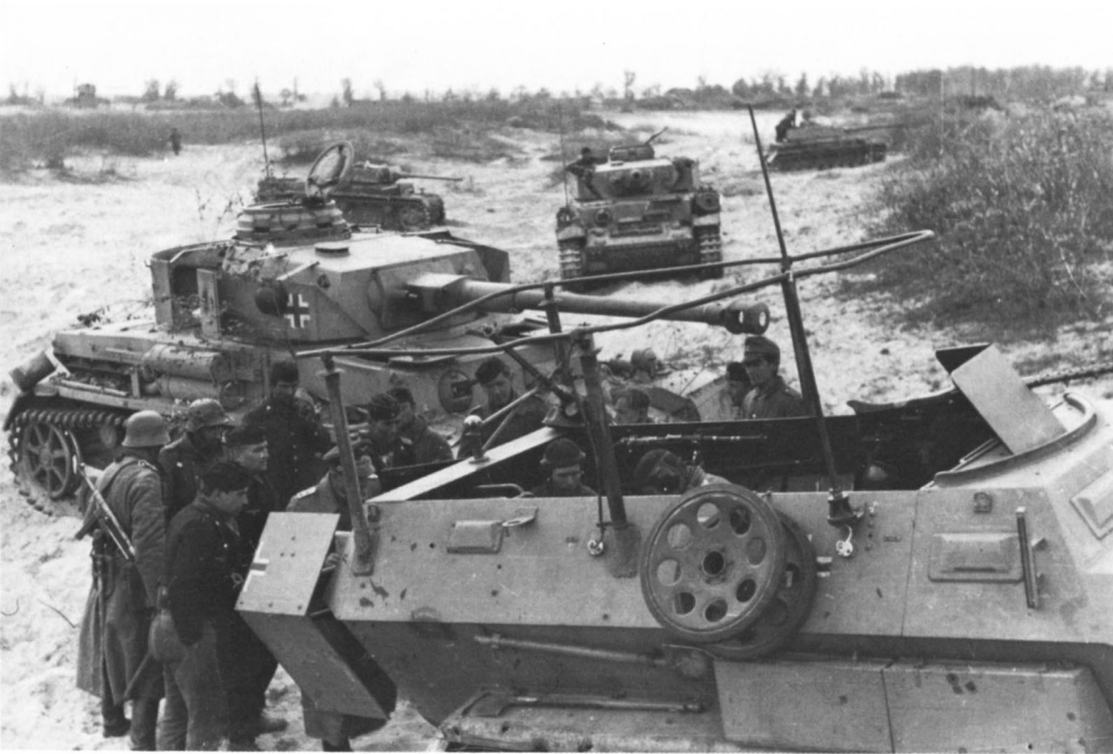
This is an early version of the ground-to-air liaison radio vehicle, the SdKfz 251/3 III. the frame aerial on this Ausf.A appears to be a field modification, as it is of an unusual design for the SdKfz 251/3. (Bundesarchiv)
