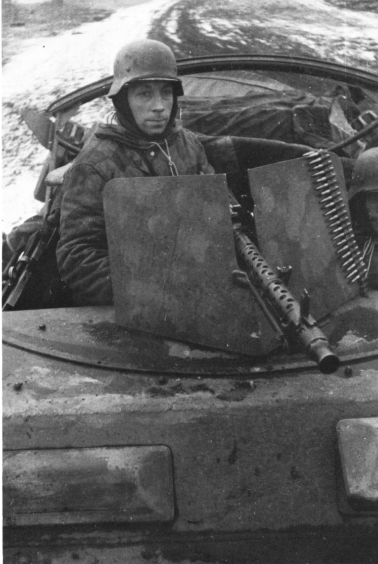
The front MG 34 mount and shield on the Ausf.B. The gun was complete with a bipod and was easily removed for use outside the vehicle. This vehicle is in the southern sector of the Eastern front, Winter 1943. (Bundesarchiv)
